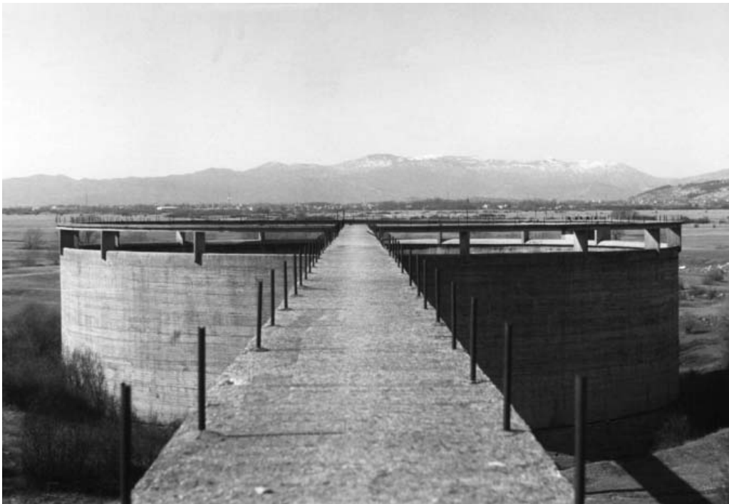
Figure 3 Photo of cylindrical dam around ponor Slivlje in the dry period.
